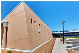
Balranald District Hospital
